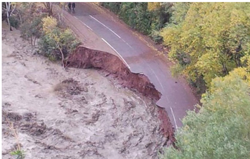
Fig. 15 Road over the Oughri river in Ouled Berhil village, 40 km from Taroudant has lost a huge part due to floods ( Source ABHSM, May 2016)
